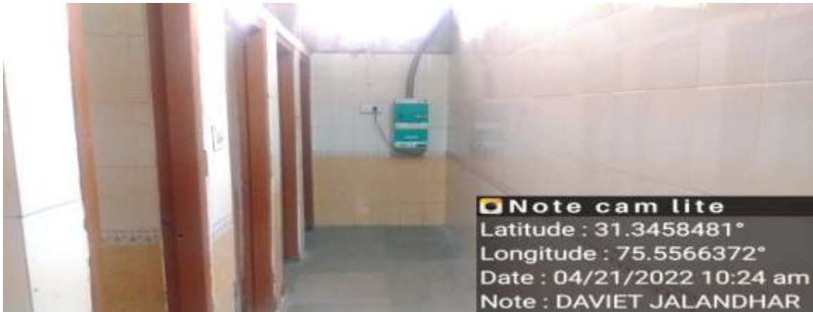
Incinerator (used for disposal of biomedical waste)
